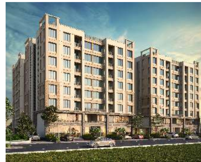
KASPER BLISS 3BHK FLATS & SHOPS @ BHAYLI
